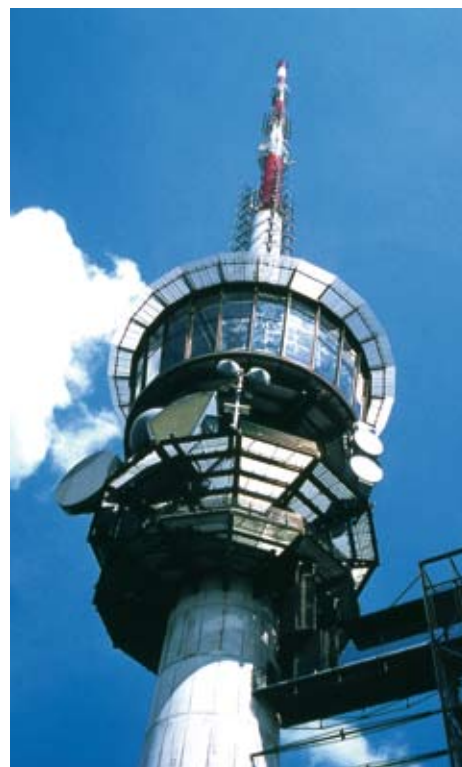
Broadcasting stations on the Rigi, canton of Schwyz (left) and Bantiger, canton of Bern (above). The directional dishes in the lower section of the towers link the station with other transmitters. The antennae for broadcasting TV and radio programmes are at the top.
